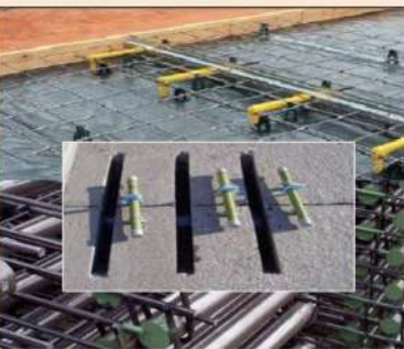
Dowel Bars Pavement Interactive
